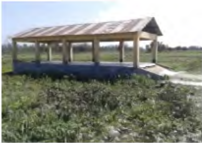
Unused Haat Shed at Jagatgaon under Matikunda –II GP, Islampur, Uttar Dinajpur
