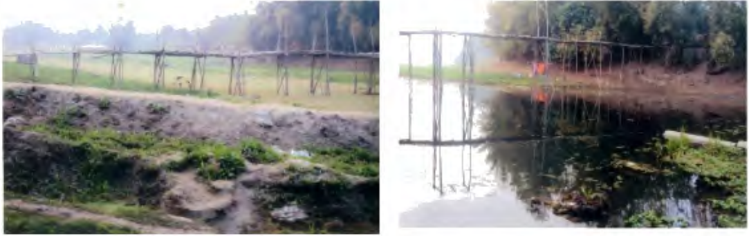
Present condition of the sites of the RCC bridges at Poolbandha (left) and Solmari (right)
