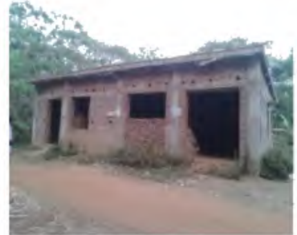
Incomplete cluster building at Kishorepur II GP, Khanakul-I Block, Hooghly
