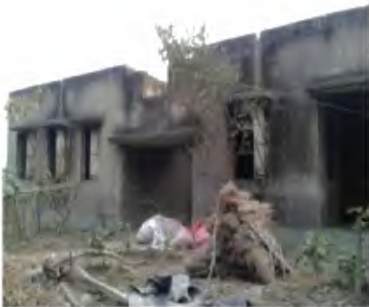
Incomplete workshed-cum-training centre at Chaltaberia under Murarisisha GP., North 24 Parganas
